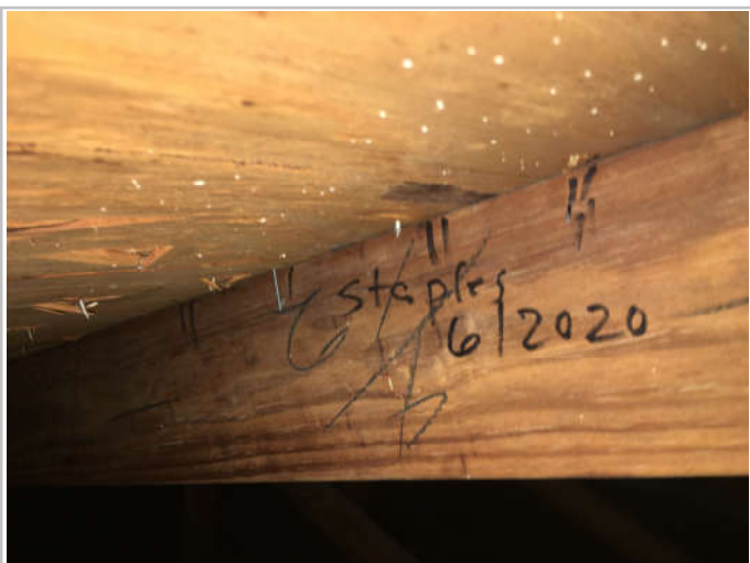
Stapled Roof Deck
